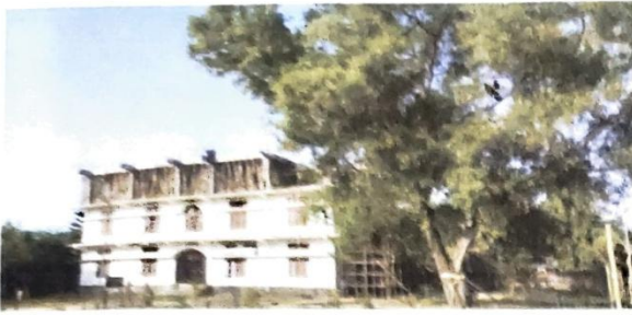
A building of the college under construction
