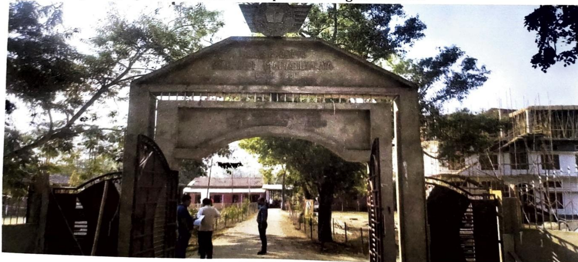
A view of the main gate of the college under construction
